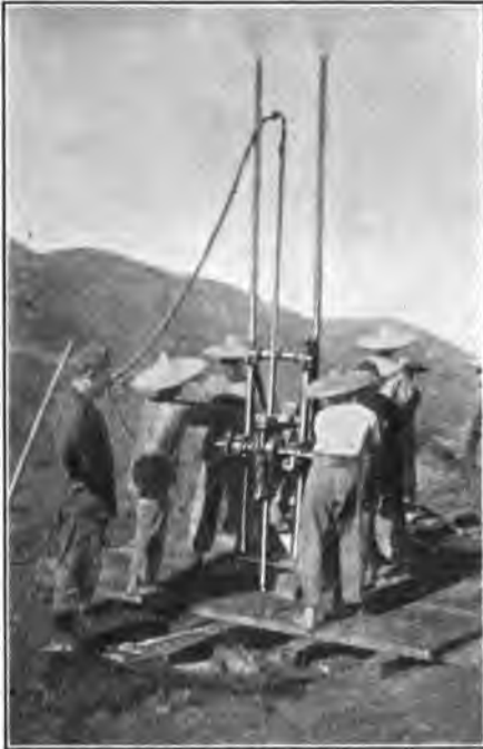
FIG. 10.—Sullivan "Bravo" diamond drill operated by coolies, North China.
